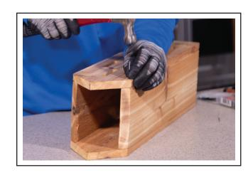
**11.** Attach the roof boards using galvanized casing nails.
