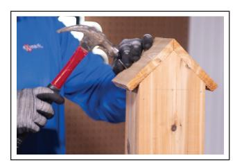
**12.** Use pliers to bend a nail in half to form the latch. Drill a pilot hole and hammer in the latch.
