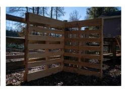
2. Next, add one of the inner pallets that will serve as a divider for each section. Secure it against the first back pallet with several screws. Be sure to offset this inner pallet when securing it to the backside. You'll need this extra surface space to attach the next middle, back pallet section to the divider.
