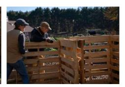
4. Finally, create removable bin gates by first cutting and fastening treated 2x4 feet to the front of the 3-bin system, then inserting 1x6 cedar boards behind each of the feet. (A total of 24 feet and 12 cedar boards will be needed.)
