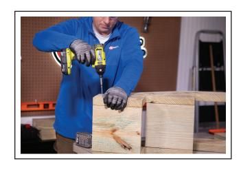
5. Take the two inside boards and slide them into the assembly, between the bottom boards and running perpendicularly with the stringers. Ensure that the edges are flush with the top and bottom of the stringers. Secure inside boards to the assembly using screws.
