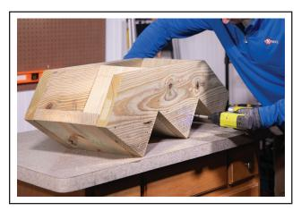
6. Take the front board and lay it over the front of the assembly, so that it completely covers the front of the bottom "step." Secure the board to the assembly using screws.
