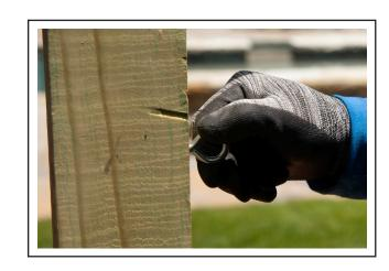
**11.** Take the wire and thread it through an eyelet. Then, take a wire rope clamp and clamp the wire.
