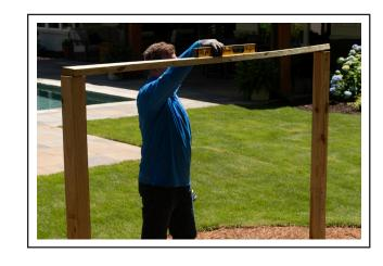
**8.** Attach the cross board to the posts using wood deck screws.
