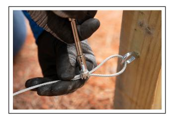
12. Pull the wire across and cut it to length, trimming off any excess. Leave an additional 3 to 4 in. of wire per cut length to attach to the turnbuckles.
