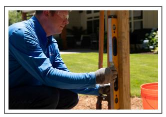
3. Add one 50-lb bag of concrete to the hole and mix with water. Let cure according to manufacturer's recommendations. Once dry, grab a shovel and fill in the rest of the hole with dirt.
