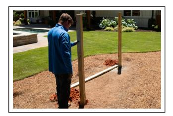
**6.** Use tamper or spare 2 in. x 4 in. board to level out the dirt around both posts.
