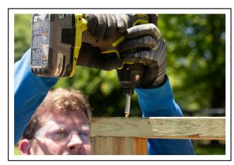
**9.** Measuring from the bottom, mark 4 points evenly spaced 16 in. from each other on the inside of both posts.
