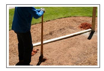
**5.** Repeat steps 1 through 3 for the other 4 in. x 4 in. x 8 ft. post, ensuring that it runs perpendicular with the ground and parallel to the already set post.
